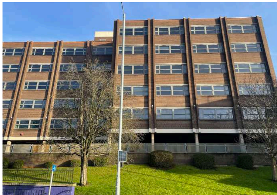
View of the building from Lower Street
