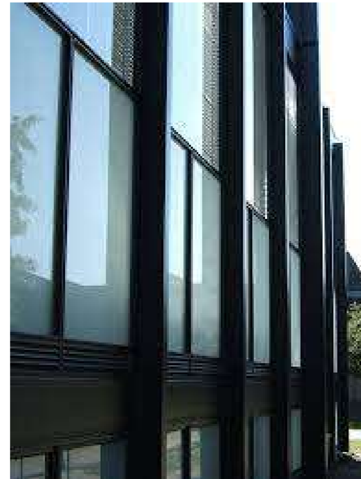
Protruding metal framework facade
