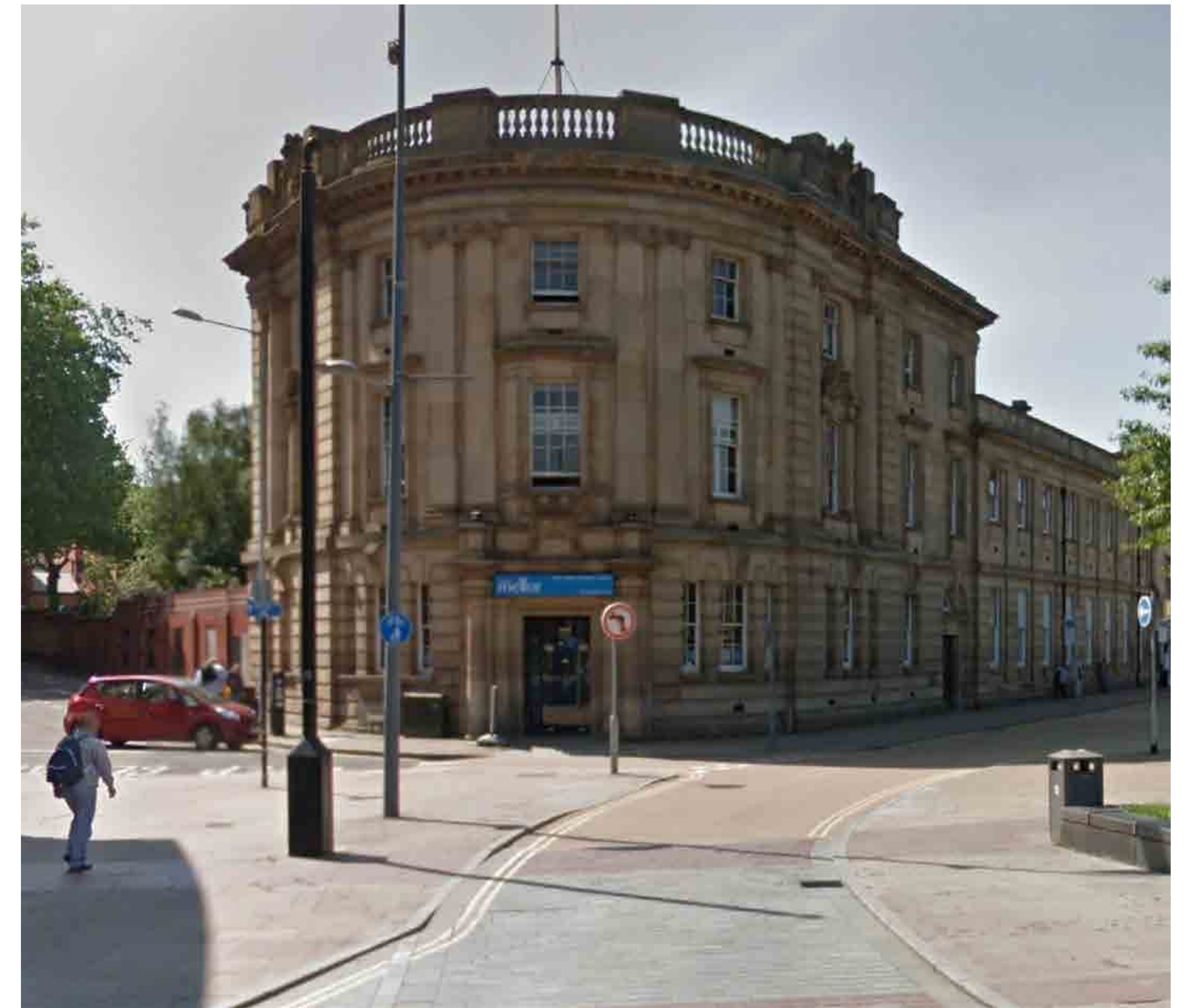
EXISTING BUILDING FROM ST PETERSGATE
