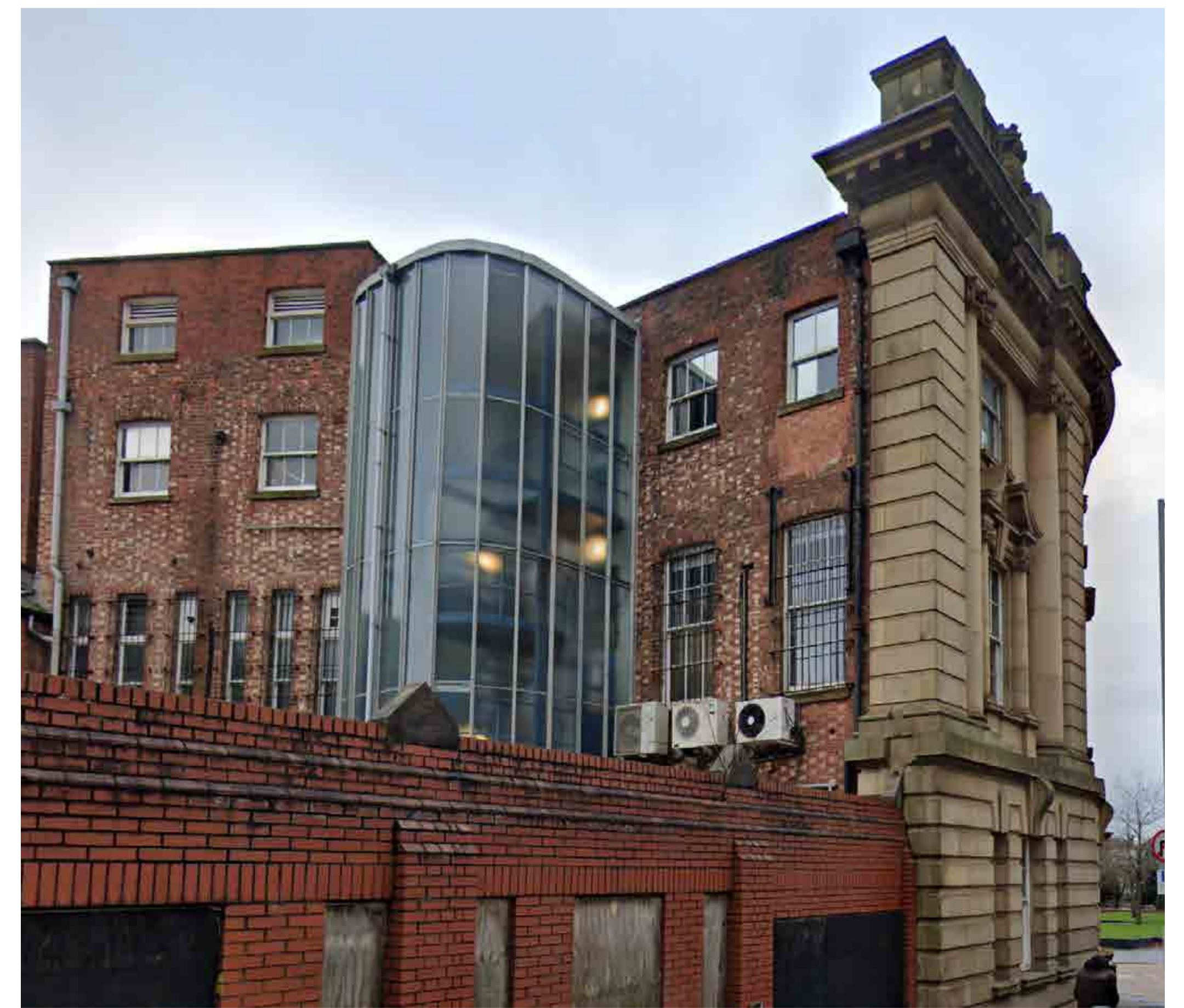
VIEW OF MODERN EXTENSION TO EXISTING BUILDING FROM LORD STREET
